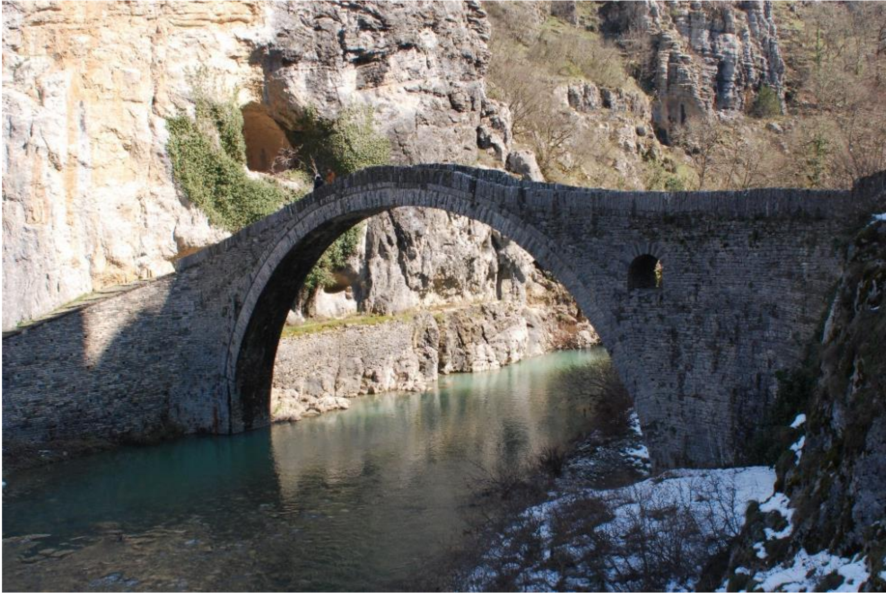
Traditional stone bridge in Greece (Voidomatis River Epirus)
